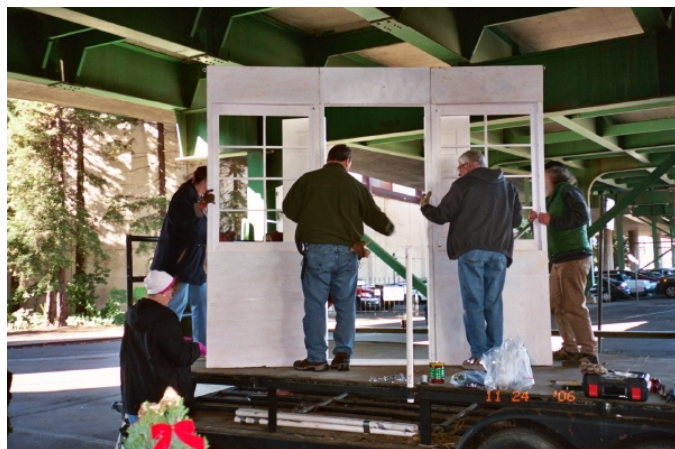
The construction crew starts the show on the road.
